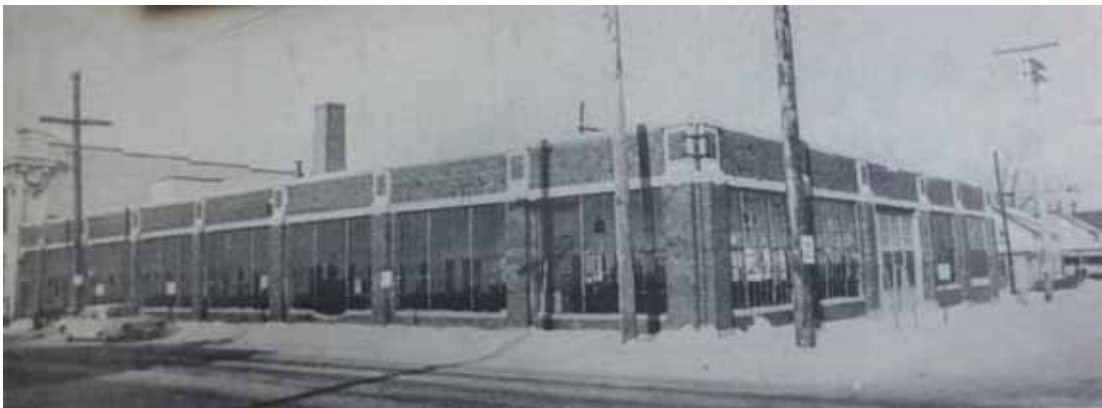
Figure 78. SSL Bus Garage before demolition, 1976 (MCPL 1976).
