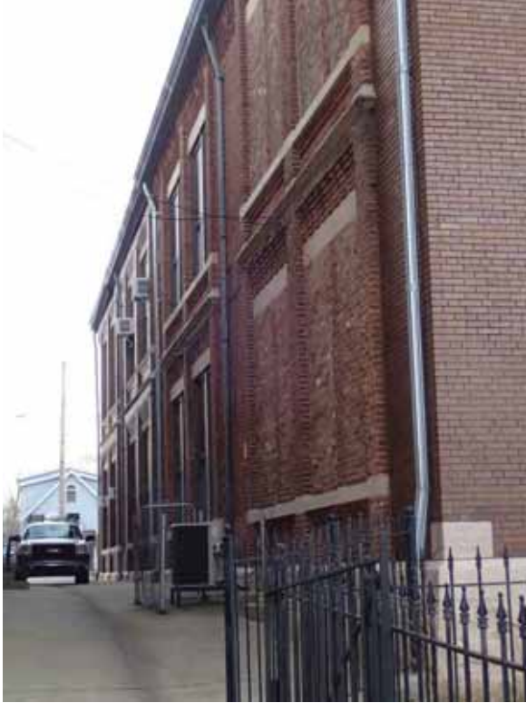
1 Figure 33. 323 10th Street (091-406-17033), detail of infilled windows on the east elevation, 2 view southwest.
