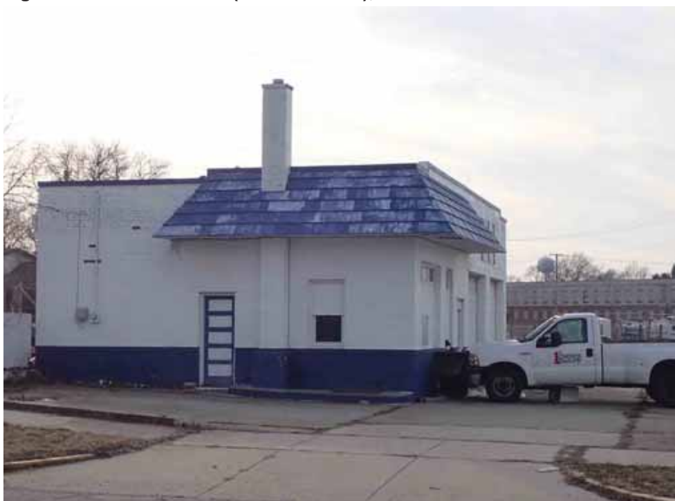
1 Figure 56. 902 11th Street (091-406-21151), view west.
