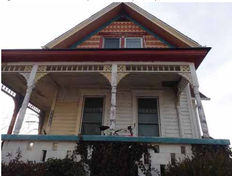
Figure 52. 1115 Ohio Street (091-406-21106), front porch detail.
