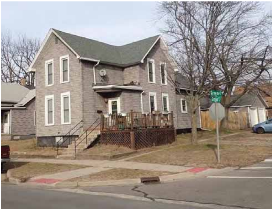
14 Figure 48. 1116 Ohio Street (091-406-21105), view northeast.
