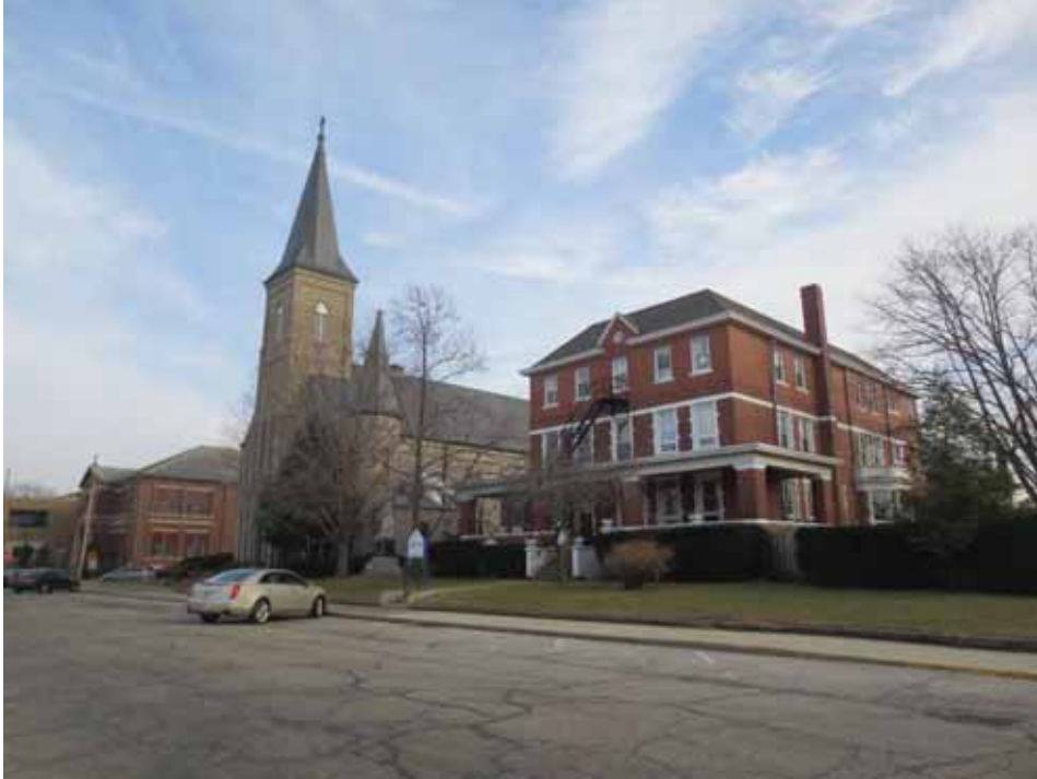
Figure 38. View southeast towards (right to left) former St. Mary's rectory/convent, church, and grade school.
