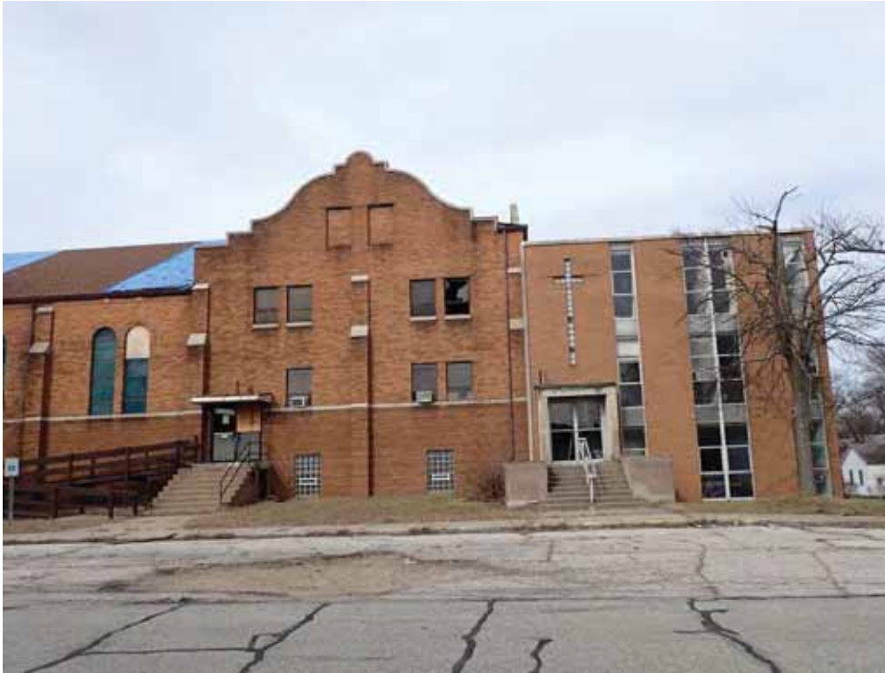
1 Figure 68. 1102 Cedar Street (091-406-21081), view north towards c. 1960 rear addition.
