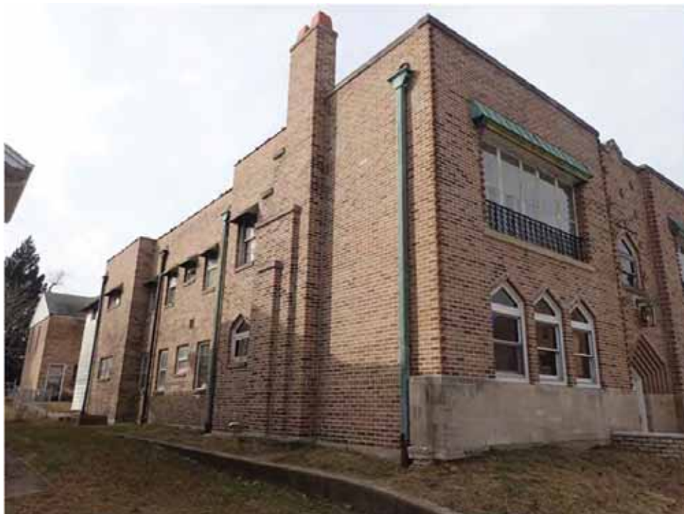
1 Figure 97. 1111 Cedar Street, view northwest. Garage visible at far left.
