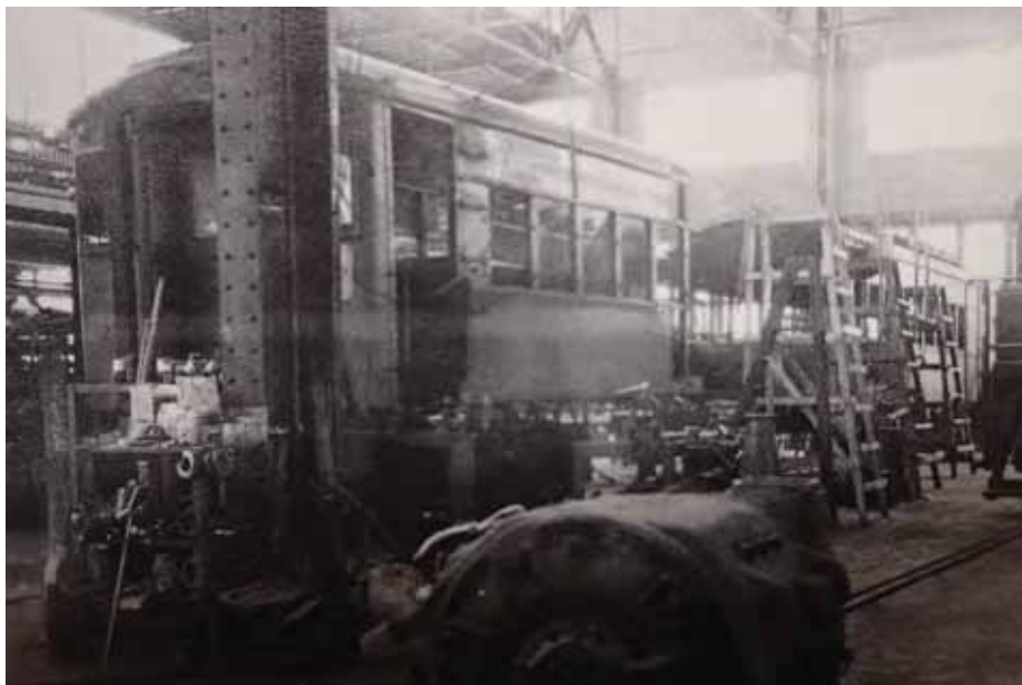
1 Figure 20. Improvements to SSL cars were undertaken locally in Michigan City shops. 2 (Top) A car is cut in half for lengthening, (bottom) new "picture" windows are installed, c. 3 1940 (Middleton 1970: 154).
