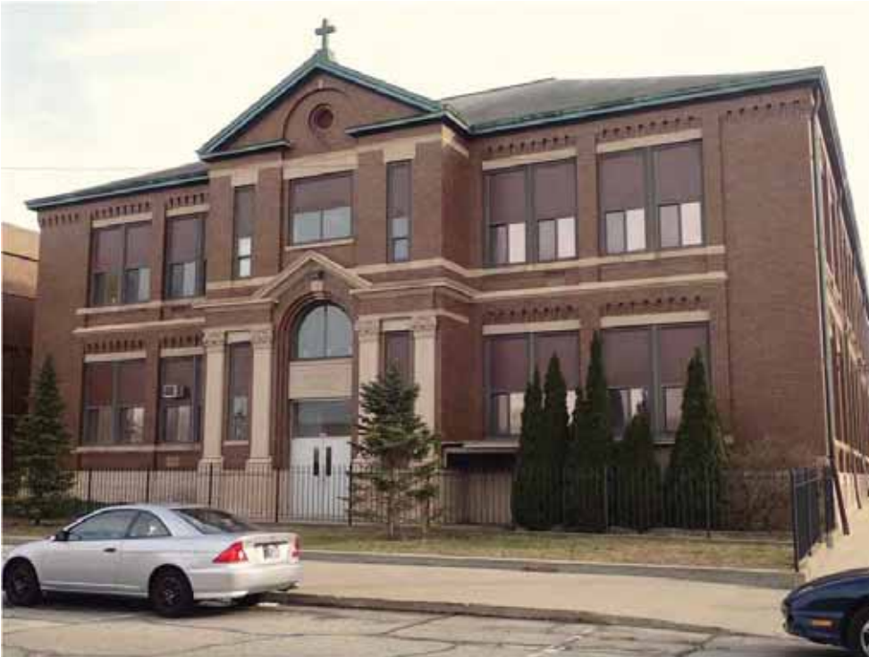
Figure 30. St. Mary's School, 323 10th Street (091-406-17033), view south.
