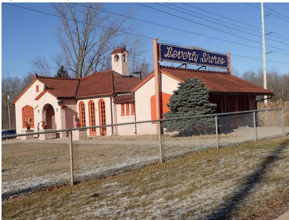
Figure 12. Beverly Shores Railroad Station (NR-0945), view north.
