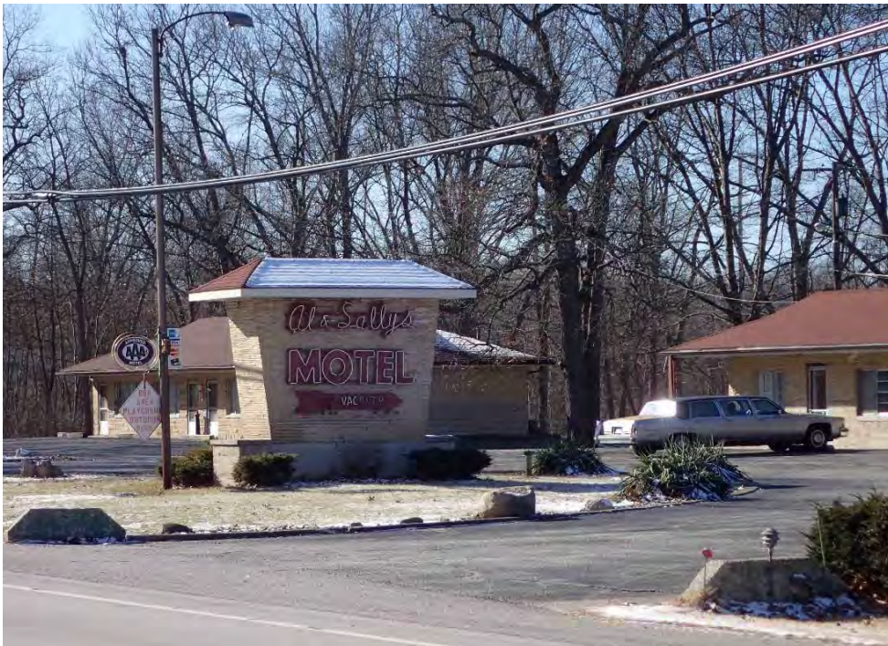
Figure 22. Al & Sally’s Motel sign, view west.
