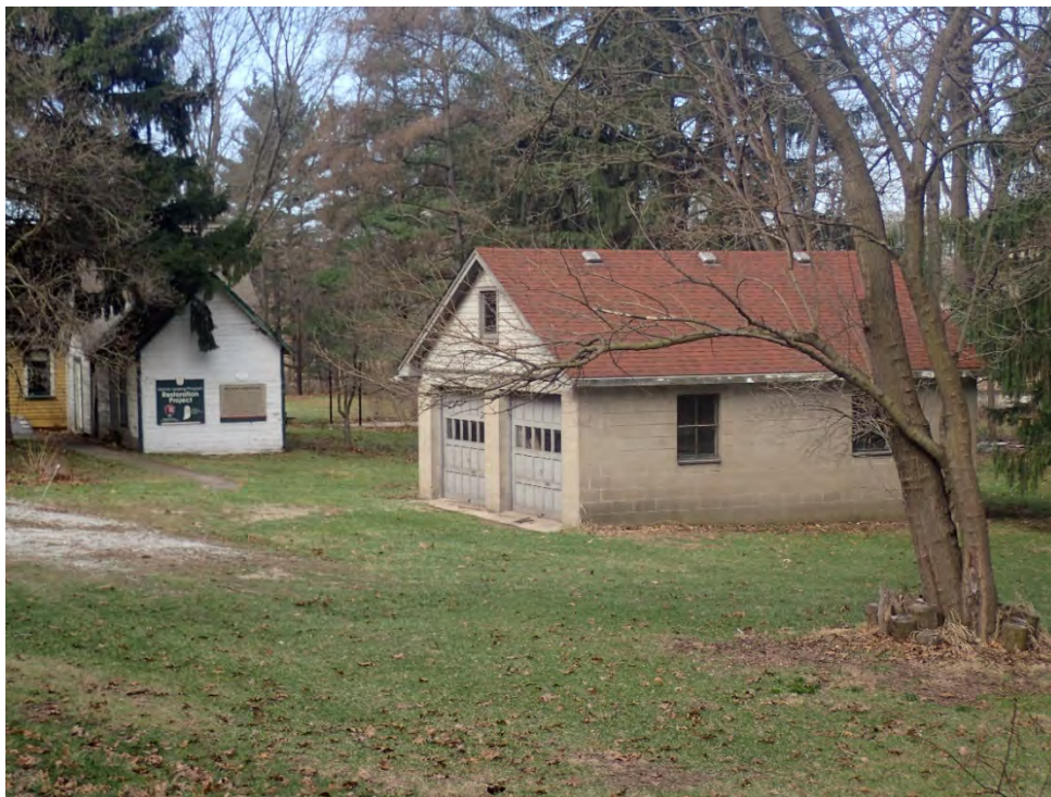
Figure 21. Oscar and Irene Nelson Farmstead (127-175-05015), garage (right) and outbuildings, view northwest.
