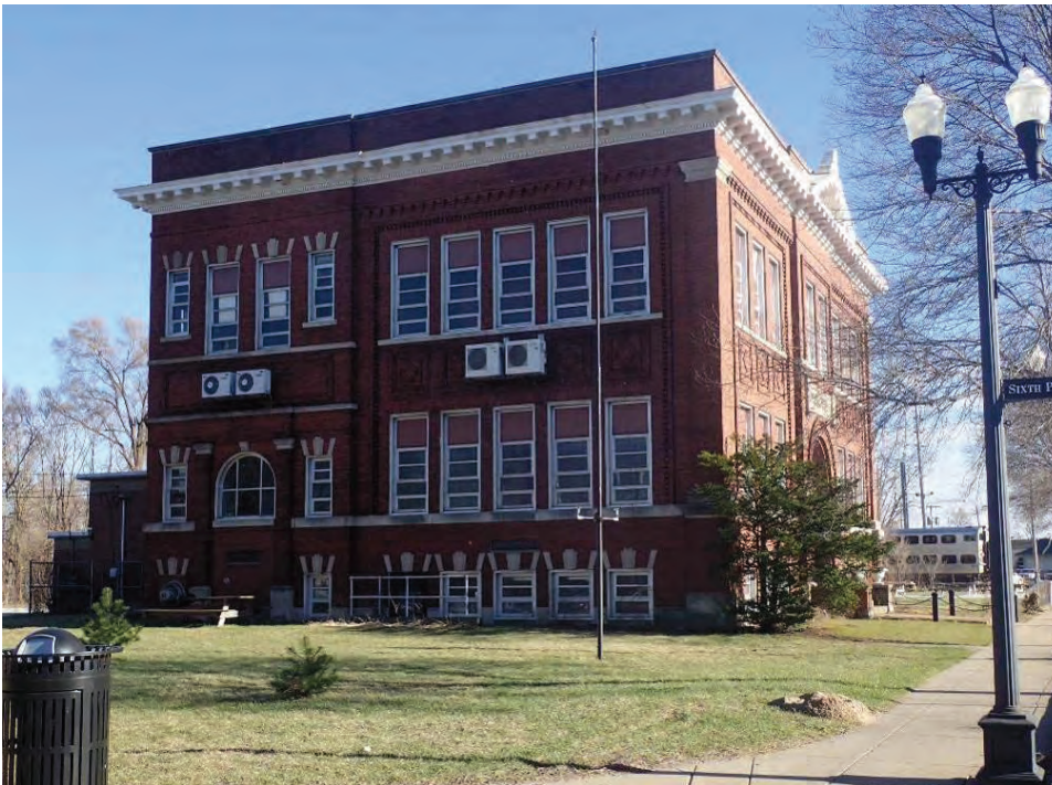
Figure 22. Miller School, view south. SSL train visible in background.
