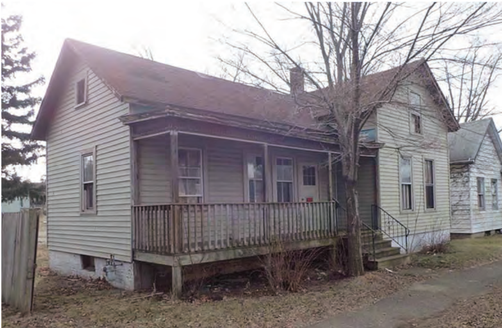
Figure 47. 505 11th Street (091-406-21080), view southwest.
