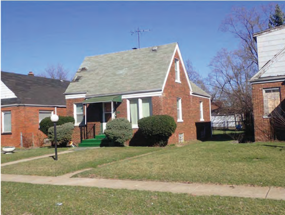
Figure 31. 637 Indiana Street (089-232-19674), view northeast.
