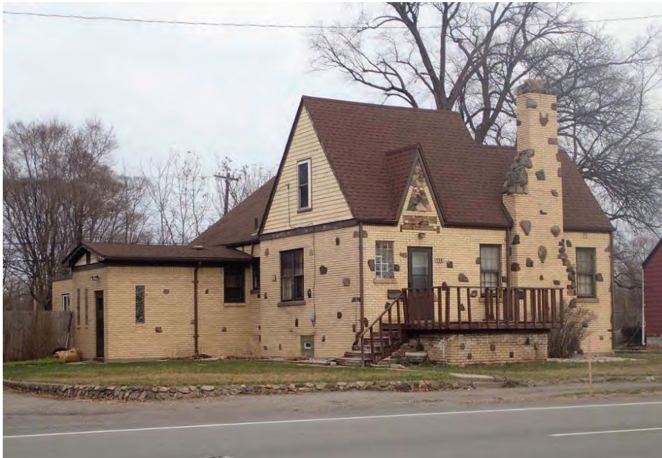
Figure 24. 5512 E. Melton Road, view northeast towards façade.
