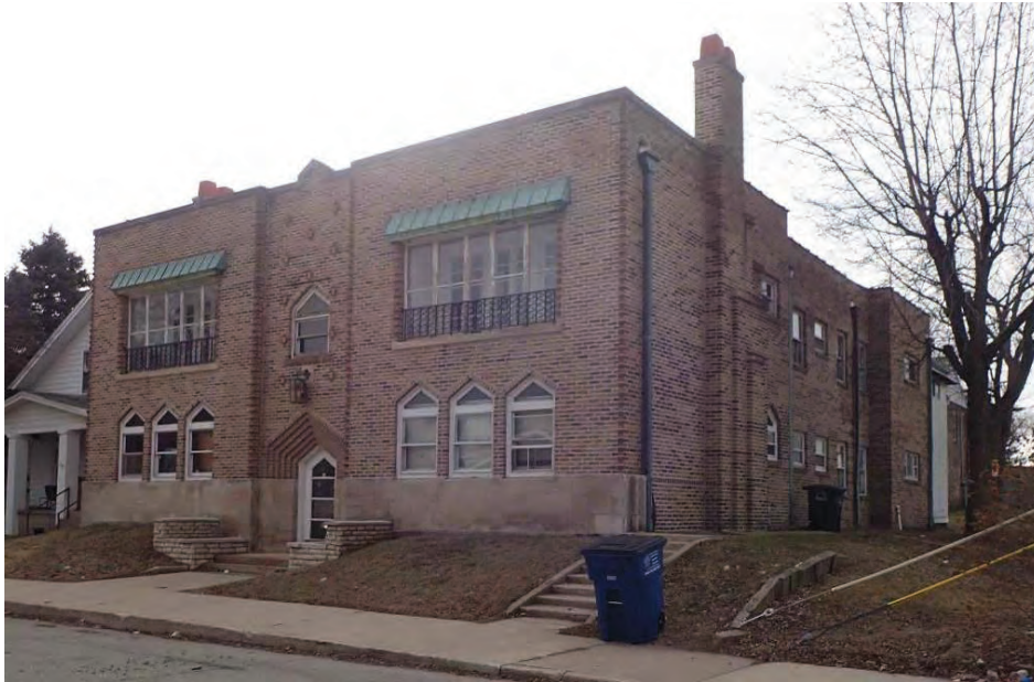
Figure 14. Behrnt Flats, view southwest towards façade.
