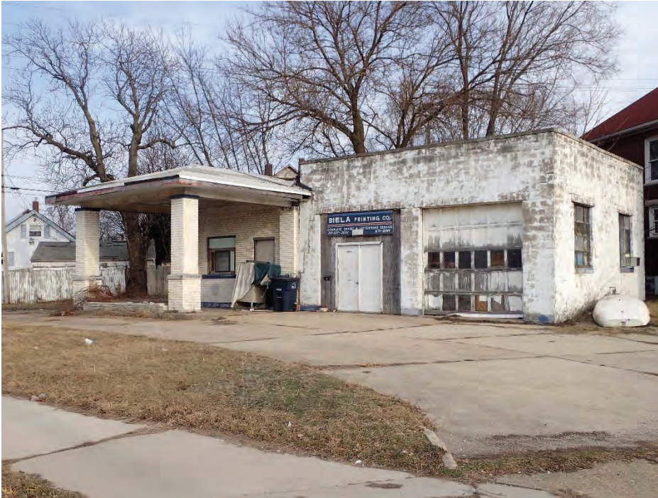
Figure 10. Commercial Building, 1004 Kentucky Street, view southeast.
