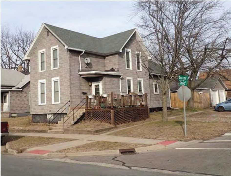
Figure 8. 1116 Ohio Street (091-406-21105), view northeast.
