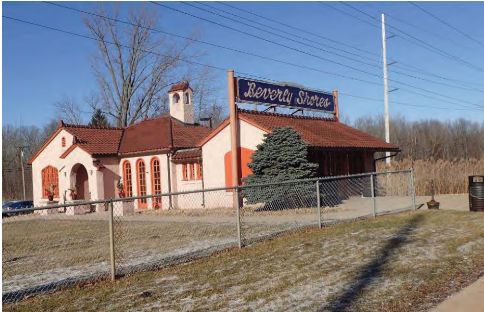
Figure 17. Beverly Shores Station, view northeast; platform to the right.
