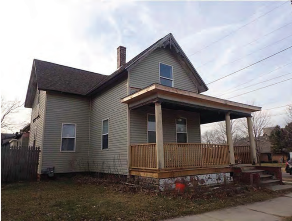
Figure 7.1101 Elston Street (091-406-21103), view northwest.
