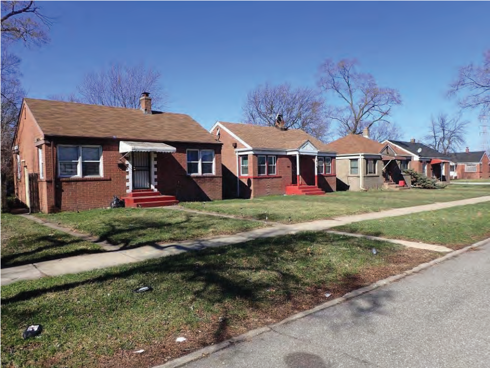
Figure 26. Hiway Homes: view northwest along Louisiana Street.
